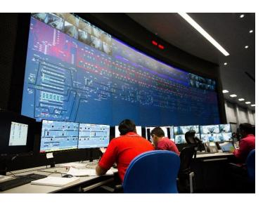
Klang Valley MRT Line 1 (Kajang Line): Design, supply, installation and commissioning of fullyautomated Cityflo 650 control system for the 51km line in the greater Kuala Lumpur area spanning 31 stations. Also provided onboard equipment for 58 trains and 16 maintenance vehicles. Offering passengers safe and efficient travel within 90 minutes between the north-west and the south-east of the city since December 2016.
