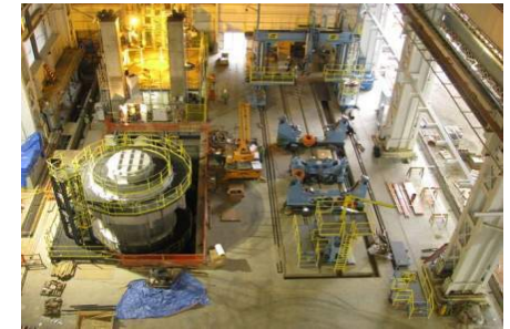
Chattanooga turbines factory (USA): inauguration in June 2010
