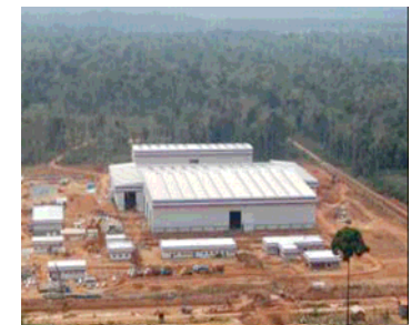
IMMA hydro factory (Brazil) inaugurated in April 2010
